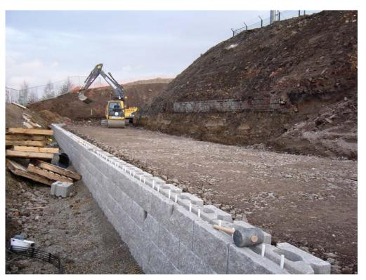
PSA Design were commissioned by Tesco to design an 8m high retaining structure for a new store development in Bradford. Two reinforced soil walls were proposed on the site to support a Service Yard and to support the car park along its Northern and Eastern boundaries.
