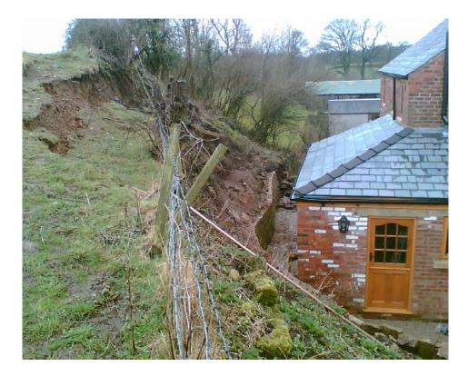
PSA Design were contacted to inspect a slope failure that had resulted in a slope adjacent to a property becoming unstable and slipping onto the home owner's land.
